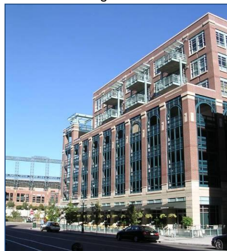
Integrated Building & Parking Structure
