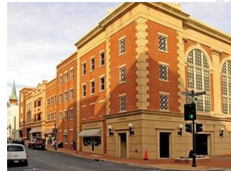
Brick Parking Structure with vertical fenestration
